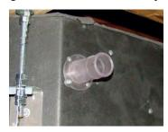
The cassette unit comes with a grey connection hose with clamp. This hose is connected to the cassette assembly discharge hose port. The other end of the hose is sized to accept 3/4 " PVC piping.
