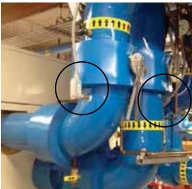
Figure 15 - Flow Sensors (DPT)
