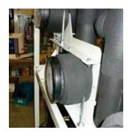
With gasket in place on each header of the positioned unit (see Figure 11), move the second module into position and line up the piping. Ensure alignment is maintained for any additional modules to be added.
