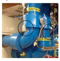
Figure 15 - Flow Sensors (DPT)
