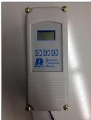
**Liquid Solution Temperature Control:** The liquid solution temperature control is an adjustable, microprocessor-based temperature control. This control receives temperature information from a thermistor located on the liquid solution supply line. A liquid crystal display continually indicates the liquid solution temperature. The control is mounted inside the chiller cabinet.
