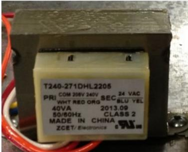
**Control Transformer:** The control transformer is rated at 24 vac, 40 va (1.6 amps @ 24vac).
