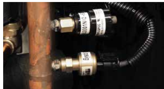
Figure 41 - Discharge Pressure Transducer
