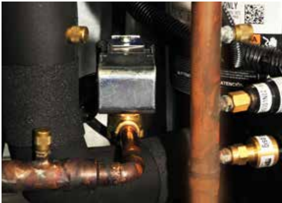
Figure 43 - Solenoid Valve
