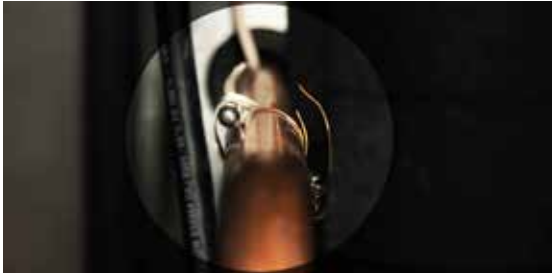
Figure 42 - Defrost Temperature Sensor
