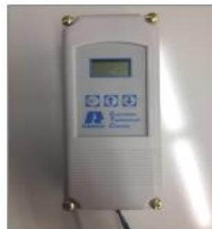
**Liquid Solution Temperature Control:** The liquid solution temperature control is an adjustable, microprocessor-based temperature control. This control receives temperature information from a thermostat located on the liquid solution supply line. A liquid crystal display continually indicates the liquid solution temperature. The control is mounted inside the chiller cabinet.
