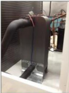
**Brazed Plate Heat Exchanger:** The heat exchanger (or evaporator) is of a brazed copper and stainless steel design. Refrigerant and liquid solution are channeled through the narrow openings between the plates and flow in opposite directions. The counter flow design and fluid turbulence ensures maximum heat exchange at minimal pressure drops.
