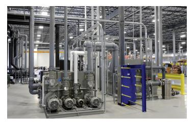
Thermal Care offers an extensive line of pre-engineered systems for air-to-water heat exchanger or cooling tower applications. Our reservoirs come in stainless steel or fiberglass with a powerful PLC control system for single point operation of chilling and towers systems. A heat exchanger is available for a closed loop system to isolate the quenchant from the coolant to reduce operating and maintenance costs. Outdoor duty systems are also available.
