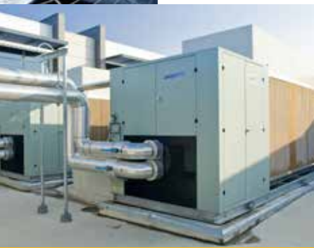
Use of evaporative pre-cooling to minimize air-cooled power consumption is very efficient from an operating cost perspective.
